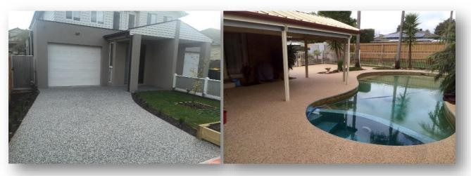
Astro's Porous Pebble Paving is a low maintenance product that is ideal for pathways, driveways and can be installed over existing surface without any demolition works.
